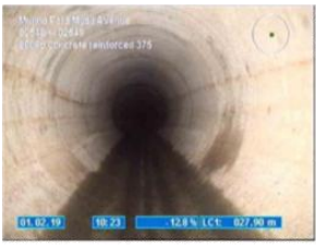
Pipe in good condition
