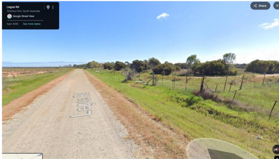
Figure 2-2 Existing Legoe Road, with subject site to the right
