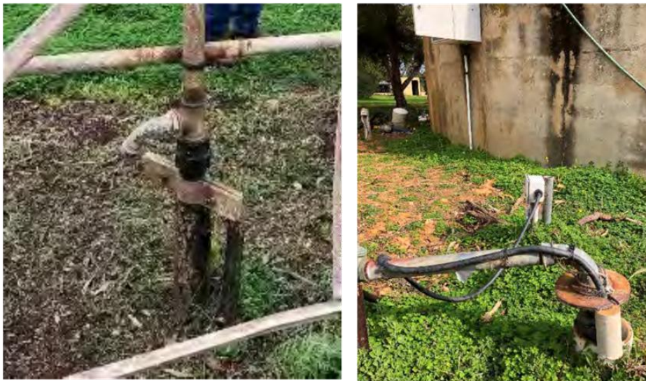
FIGURE 5-3 UNUSED 37 M DEEP WINDMILL WELL 6528-248 ACCESSING THE QUATERNARY AQUIFER AND THE 96 M DEEP T1 WELL 6528-2039 (TESTED)
