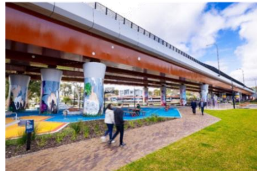
Urban realm improvements as part of the Ovingham Level Crossing Removal
