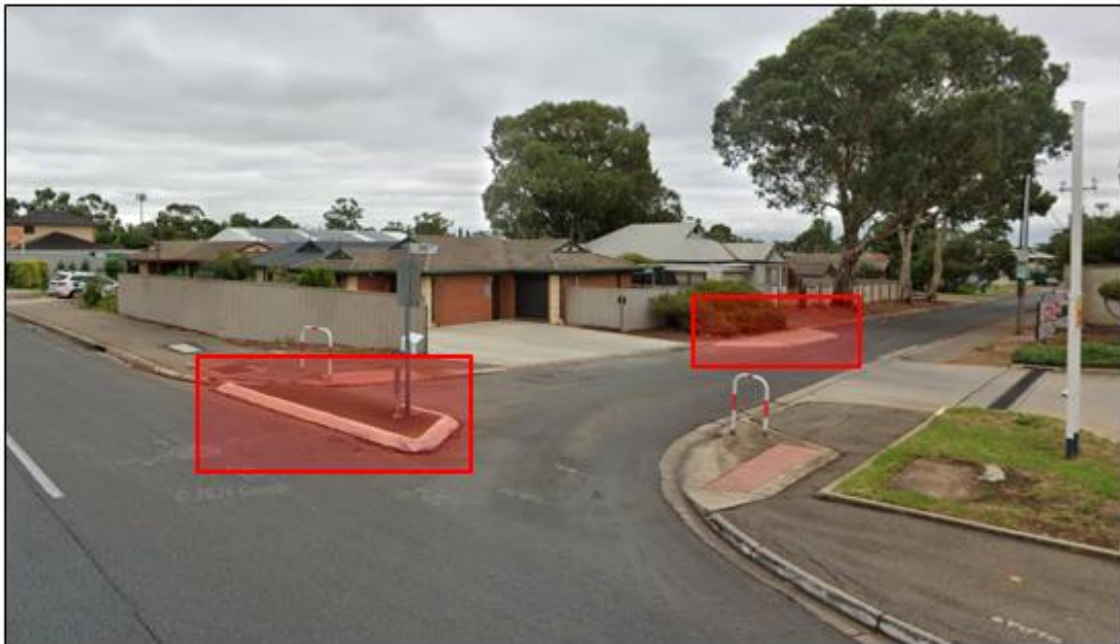
Figure 6 – Raised islands precluding left-in access to Jane Street from Main North Road.
