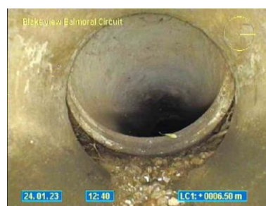
Pipe requiring renewal works
