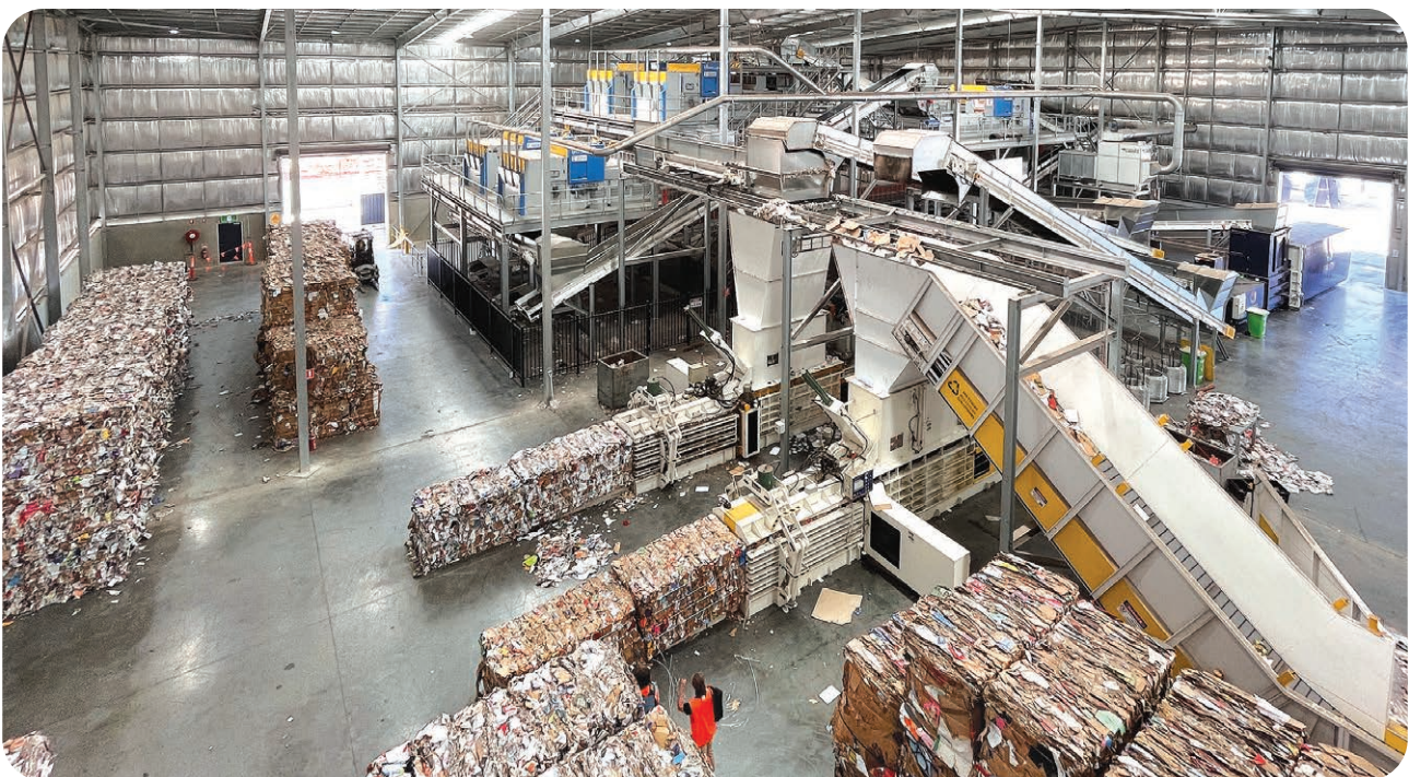
NAWMA's Material Recovery Facility (MRF) processed 44,000 tonnes this year.
