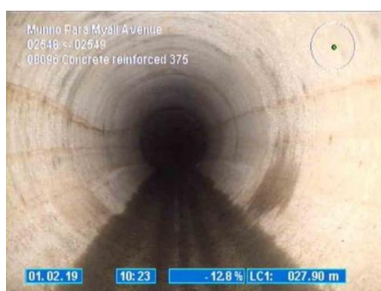
Pipe in good condition
