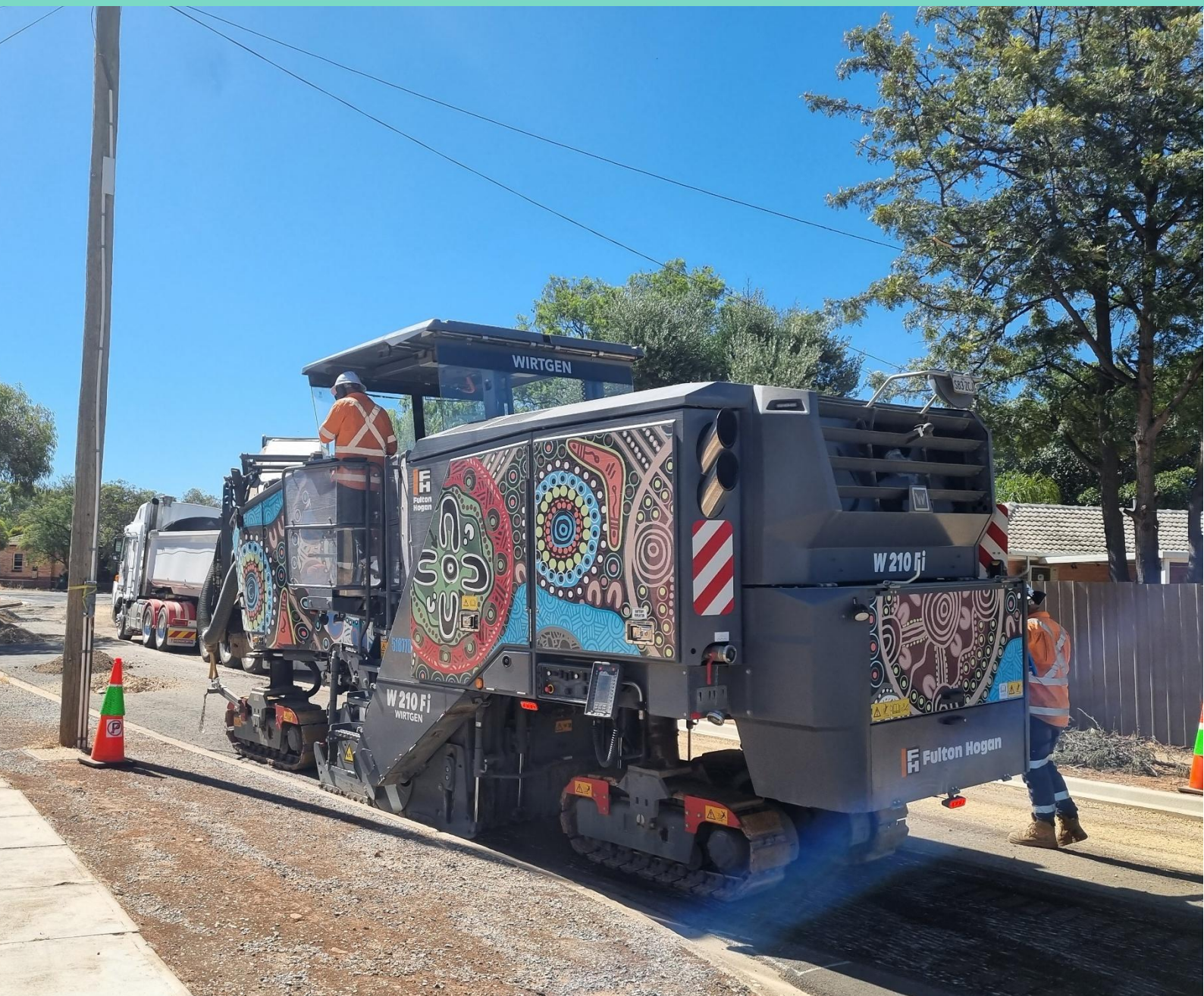
Chillingworth Road, Elizabeth East road resurfacing
